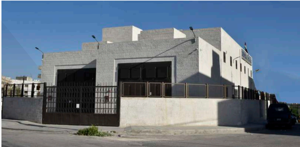
Shafa Badran Main Substation, 2022.
