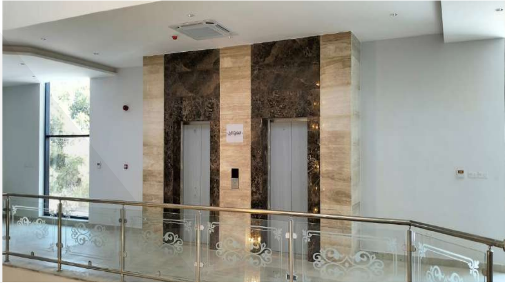
Construction of an Army Hotel (Royal Jordanian Command and Staff College), 2024.
