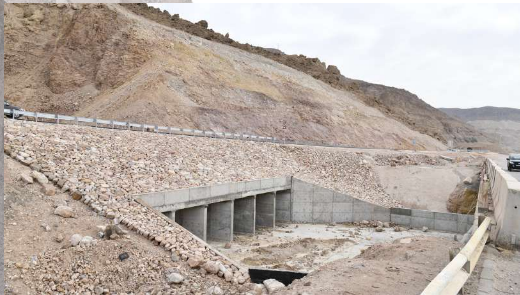
Protection Works For Bridges Along Dead Sea – Ghor Hadetha –Road –Package 2, 2021.
